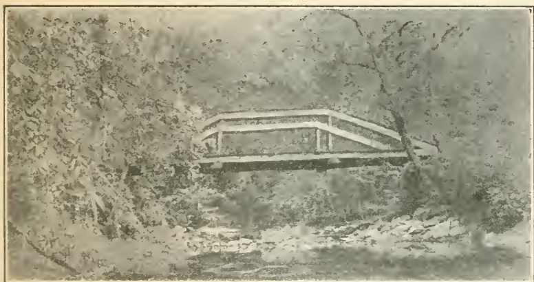
CUB RUN BRIDGE, 1910.
